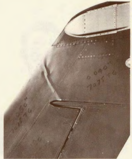
Overstress at rudder hinge caused skin buckling.
